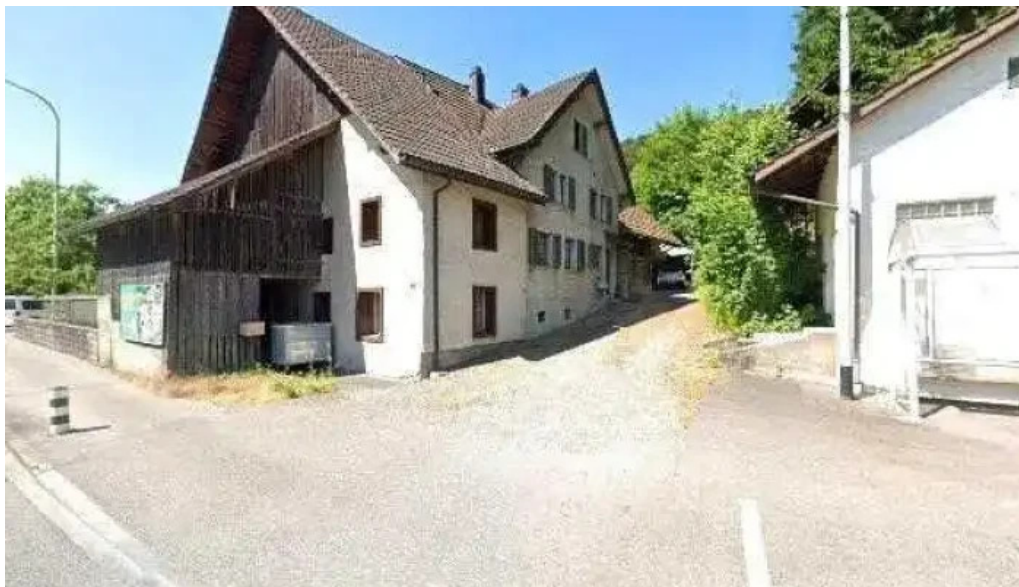
Hotel villmergen street view 360deg fotos
