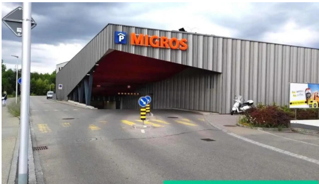
Migrol ladestation oberwil
