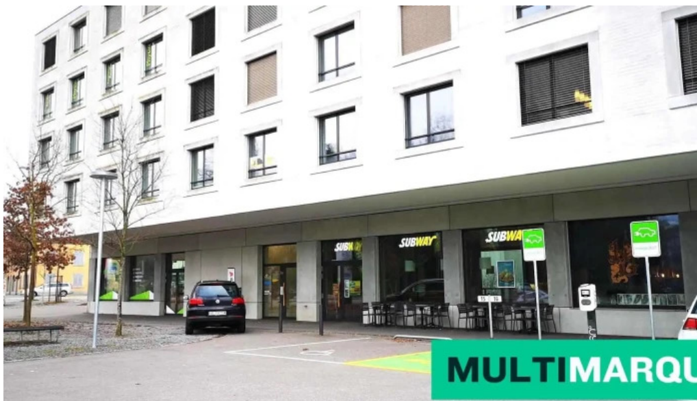
Swisscharge charging station alle
