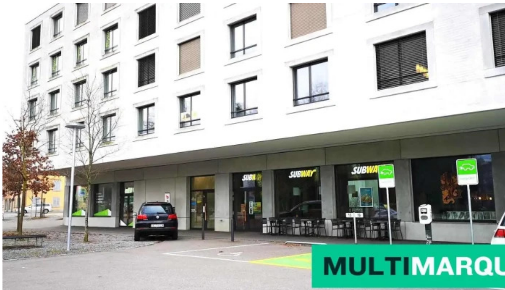
Swisscharge charging station windisch
